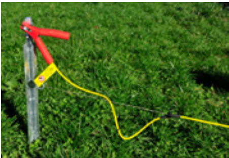
Ground connection, e.g. on the mast or with earth spike through clamp with strain relief
